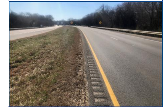
Edgeline Rumble Strips
